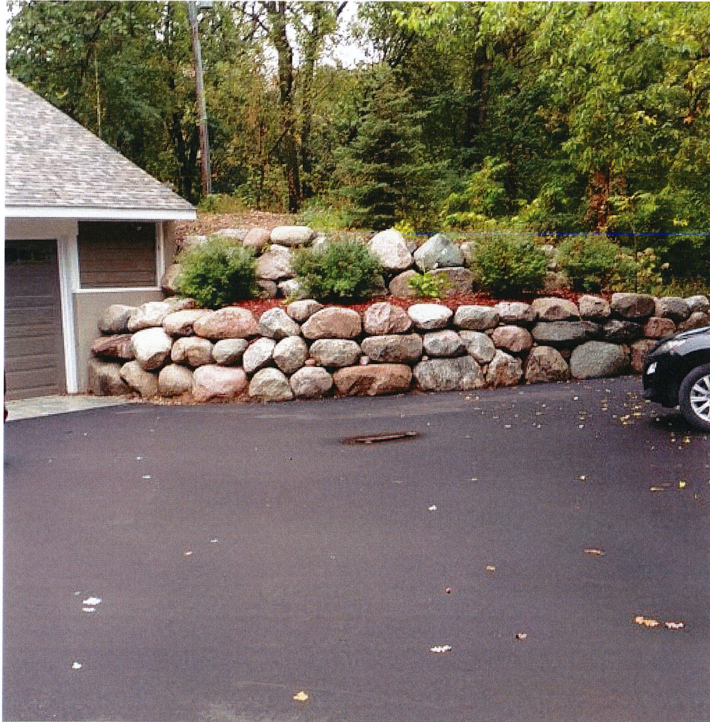
Retaining wall off of southeast corner of the garage.
