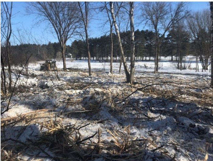
Clearing of Musser Park
